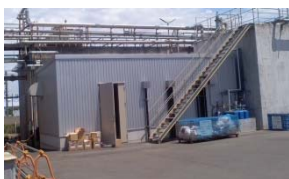
New Blower Room
